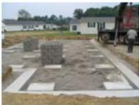
**Piers** – Piers are the most cost effective foundations, but are not available for all homes. Pier foundations involve placing concrete or other approved footers below the frost line. The footings hold the weight of the home. Then a pier, normally made of steel or stacked block supports the home between the footing and the frame of the home.
