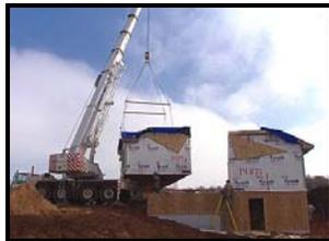
Once the home arrives at the construction site, the modular home components are craned into place and the roof is set. This is usually accomplished in less than a day.
